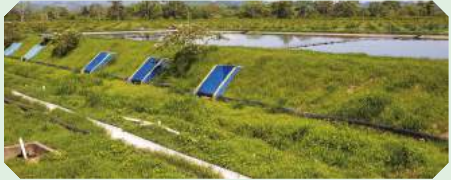
Facultative lagoon for irrigation of plantations
